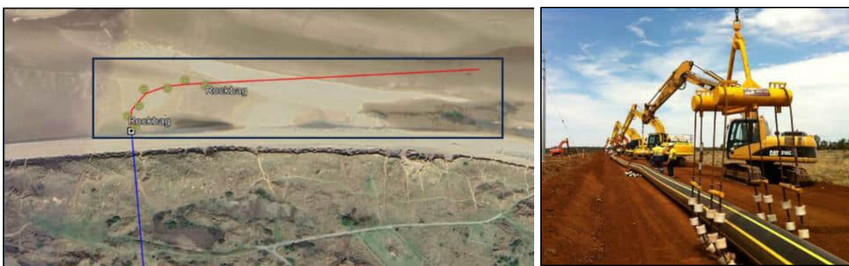
Figure 4.14: Pipe repositioned for pull back
