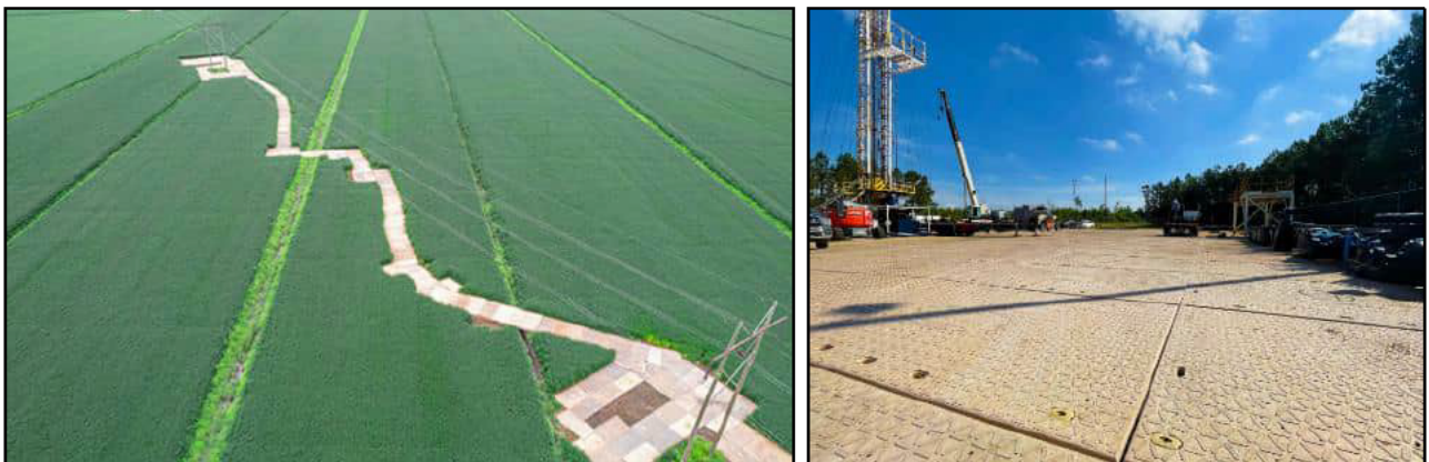
Figure 4.4: Typical temporary matting
