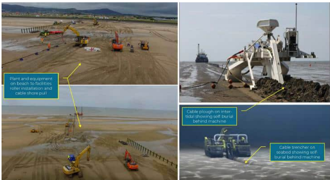
Figure 4.19: Typical plant and equipment for cable installation across inter-tidal like the offshore wind farm cables historically installed between Prestatyn and Rhyl.
