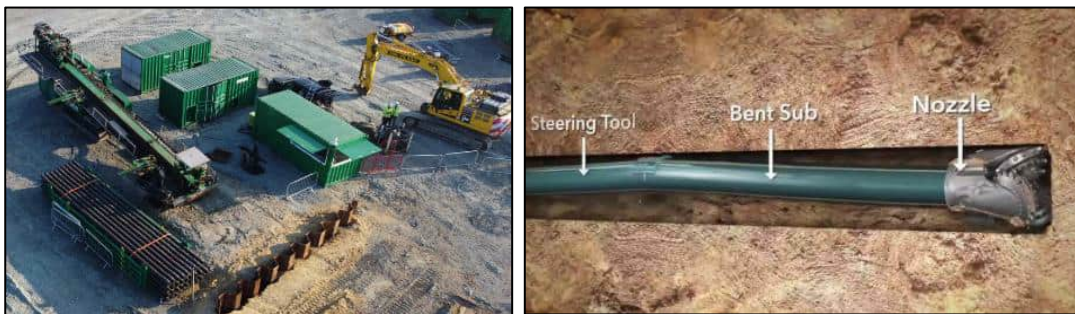
Figure 4.12: Typical drilling rig and pilot drilling assembly
