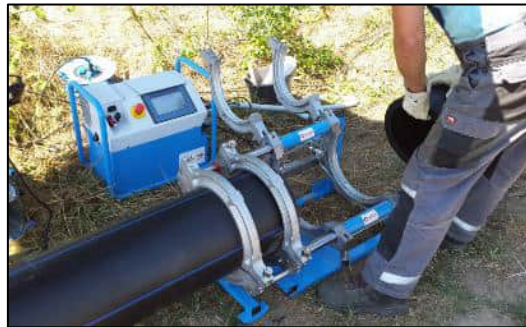
Figure 4.10: Typical pipe welding equipment, storage of pipes and welfare not shown
