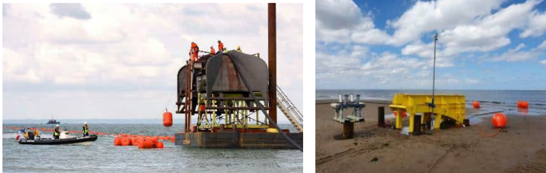
Figure 4.21: Shoreline beach chute as operated on previous projects
