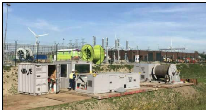
Figure 4.18: Example of typical cable pull winch
